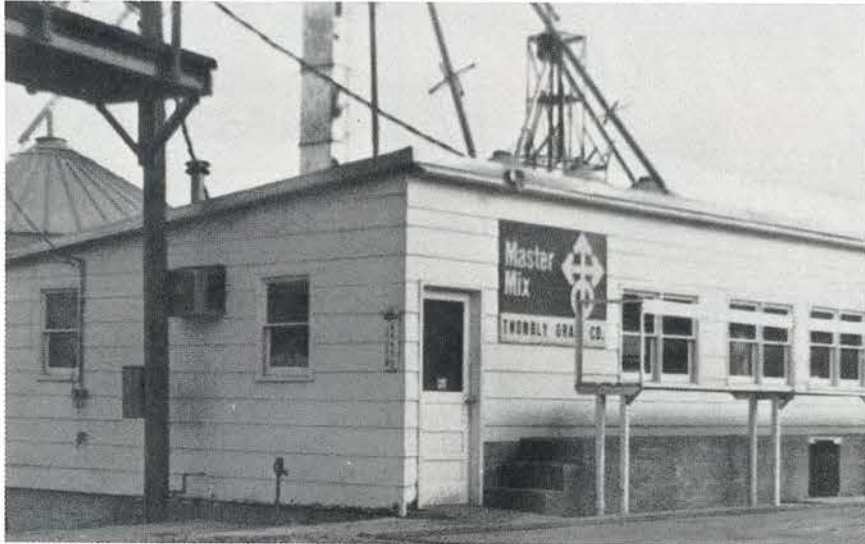
"A Full Service Elevator"
