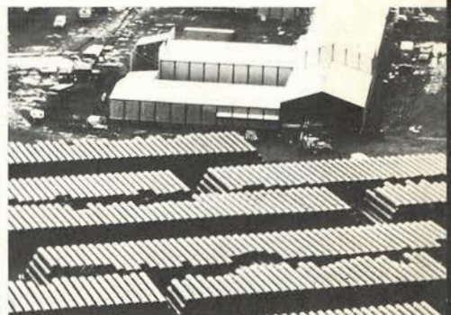
Construction proceeds on the Alaskan Pipeline with aim to eventually ease fuel crises. Photo of storage yard in Valdez, Alaska, shows a part of pipe to be used.
