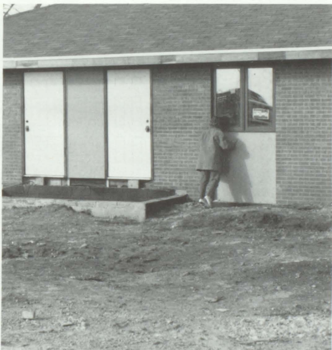
Peering into the window of the unfinished administration building, Kristi Cochren takes a sneak preview of the interior.
