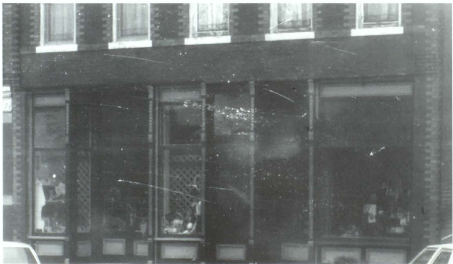
Le Coeur et Le Ame , or The Heart and Soul, owned by Debbie Simpson, is one building that was remodeled this year. Mrs. Simpson plans to turn it into a dinner theater. Photo by Chris Hoverson.
