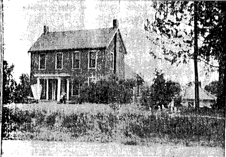
THIS 2-STORY brick house was constructed of brick made in Troy, and is among the older houses in Troy. It was originally the home of Henry Boder. It is located a block west of the public square and is now the home of Mr and Mrs Fred Worman.
