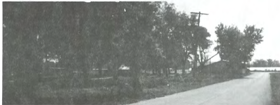
Ellsworth Trailer Court All trailers were completely destroyed.
