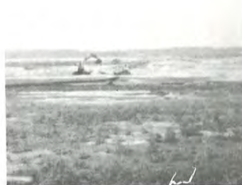
Bulldozers working at the break.
