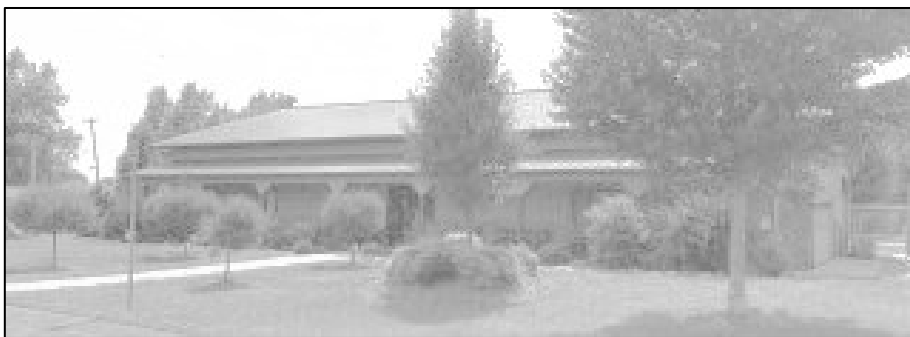
Wathena Community Building photo from Google Maps
